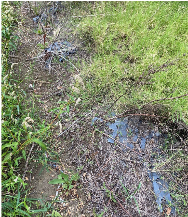
Photo 2-3. Degradation of the South Impoundment Liner
