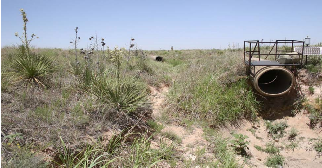
Photo 2-11. Culvert 4 (left) and Culvert 5 (right) with Erosion and Subsequent Undermining
