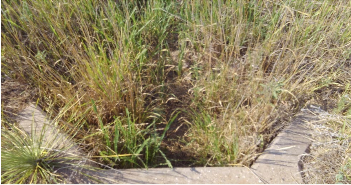
Photo 2-9. Culvert 3 in Overall Good Shape
