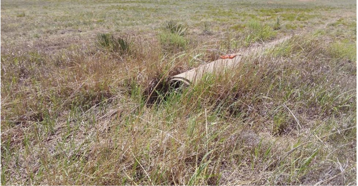
Photo 2-7. Erosion Trench at Culvert 2
