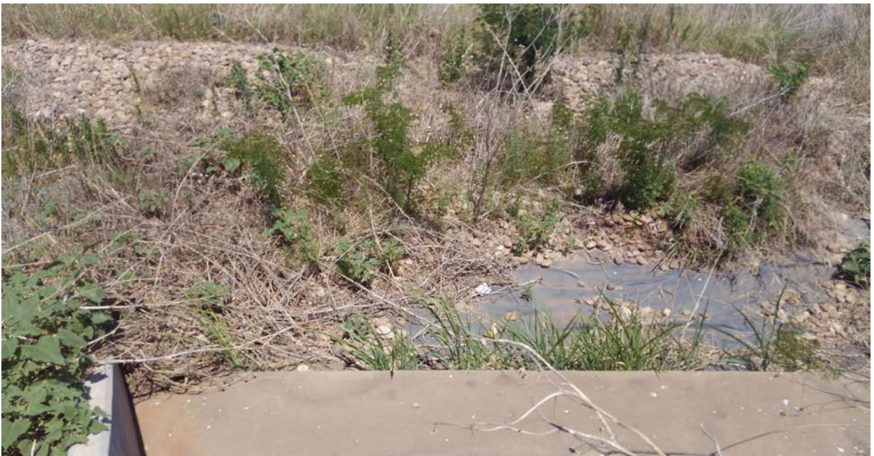
Photo 2-6. Riprap Washed Away from the Apron/Base of Culvert 1
