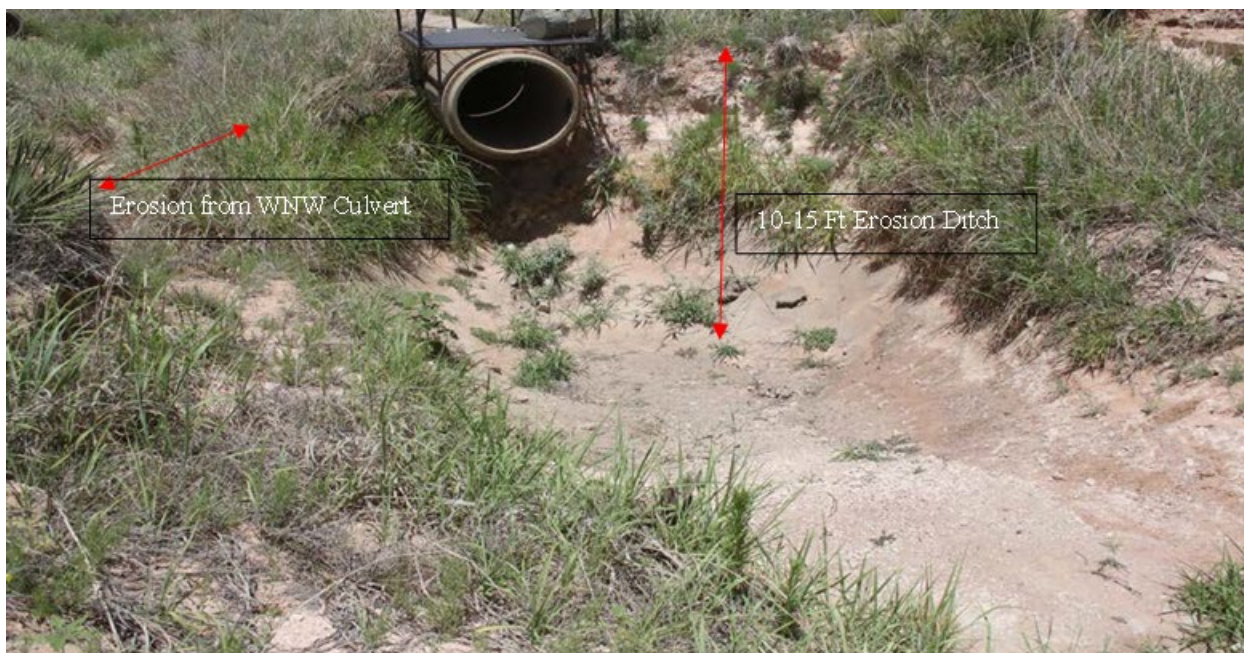
Photo 2-12. Erosion Around and Beneath Culvert 5
