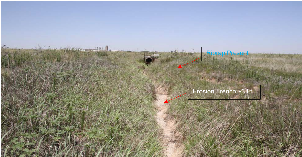
Photo 2-13. Culvert 5 and Erosion Trench
