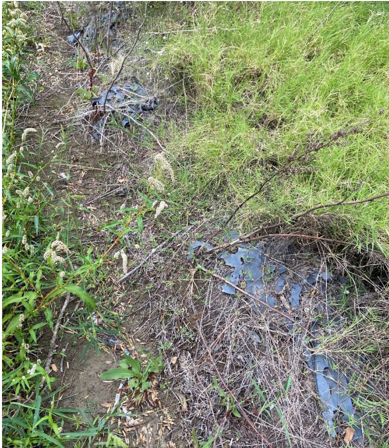
Photo 2-3. Degradation of the South Impoundment Liner
