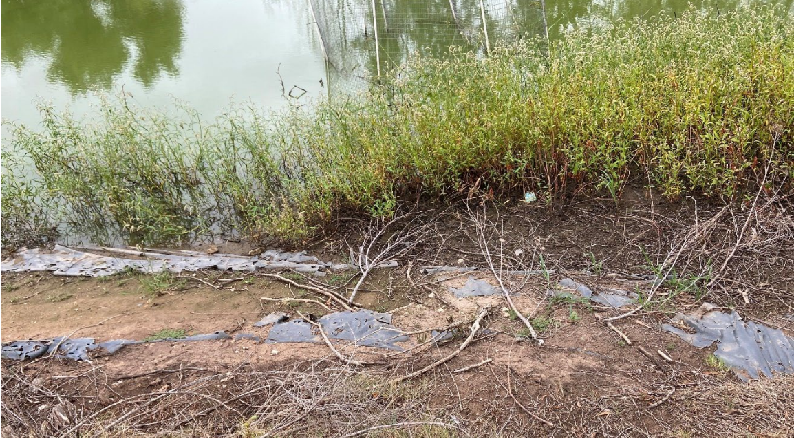
Photo 2-2. Degradation of the North Impoundment Liner
