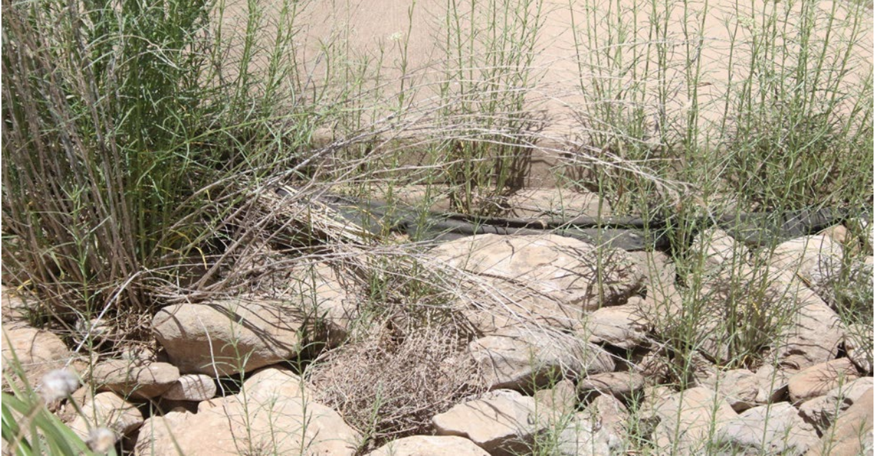
Photo 2-5. Washed-Out Riprap at Culvert 1
