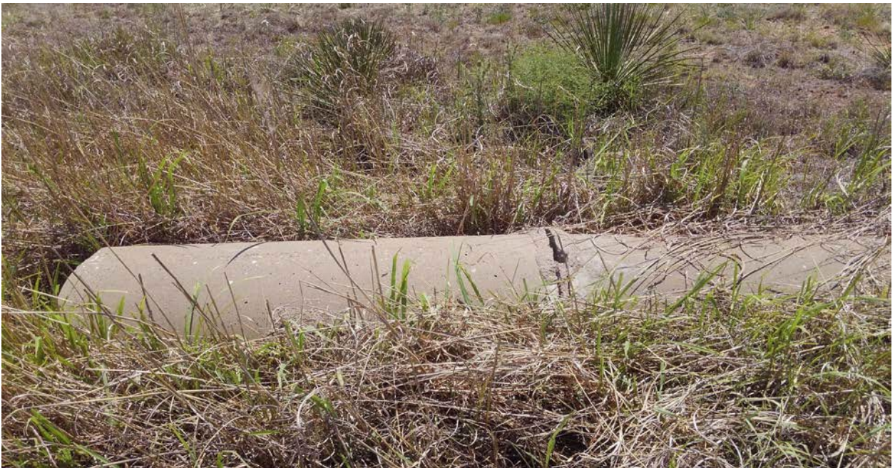
Photo 2-8. Separation in the Stormwater Line at Culvert 2
