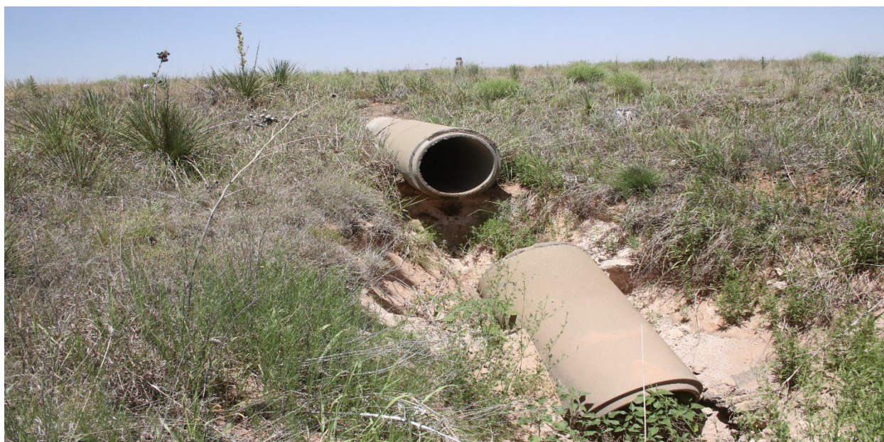
Photo 2-10. Culvert 4 Lost Section Due to Erosion and Subsequent Undermining
