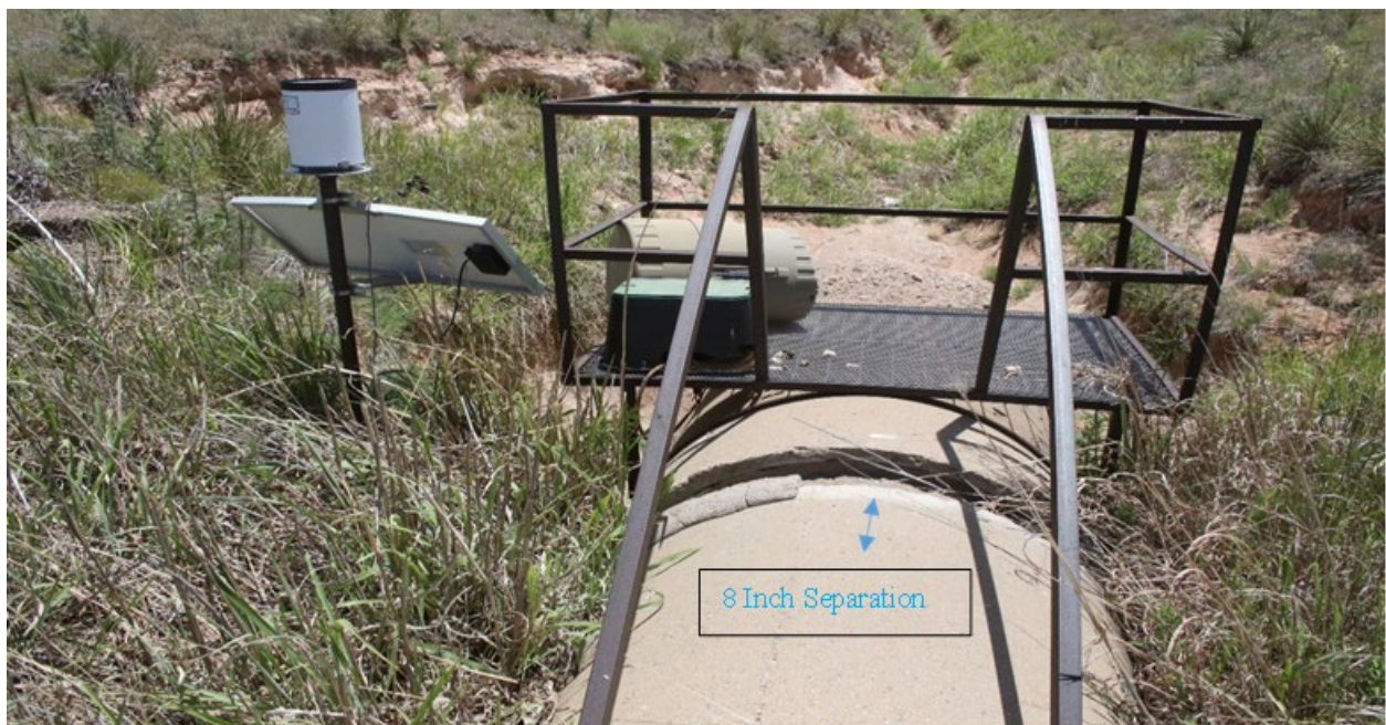
Photo 2-14. Separation in Culvert 5 Stormwater Line
